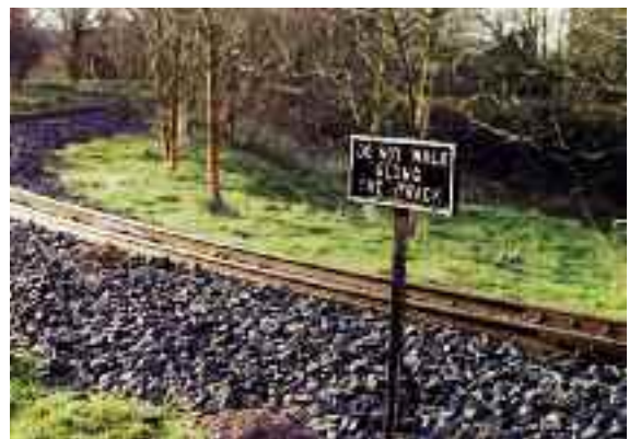
An example of ground-level track showing sleepers, fixings and ballast
